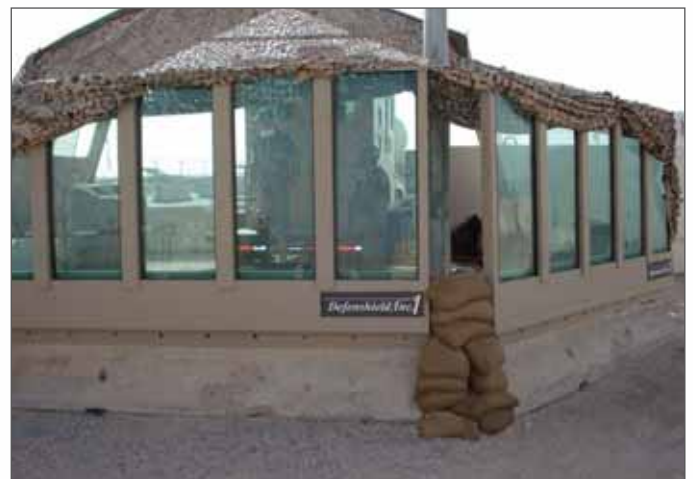
Barrier Caps in use at an Air Force FOB in Kuwait.
